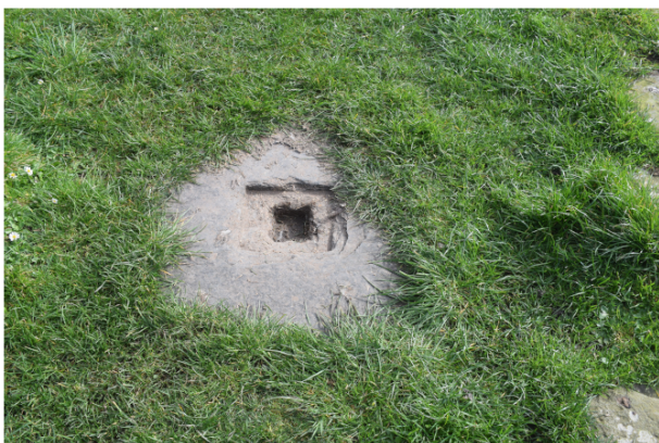
Plate 3: Mooring post footing on northern quay wall. Looking east.
